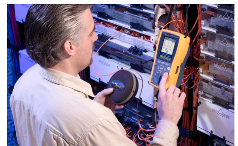
DTX with OTDR module attached and launch fiber
